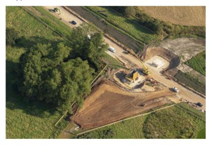
The steel shuttering has been craned into place ahead of 210 cubic meters of concrete being poured during October to form the abutments. The concrete pour will mark the largest pour on the scheme to date.
